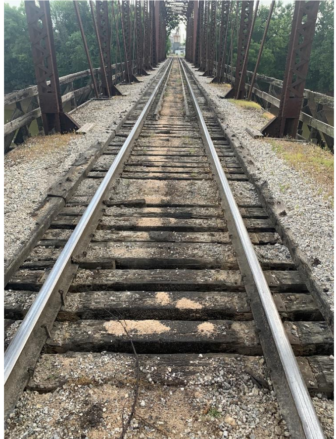
(247.4-1 Thru Truss w/Open tie deck)
