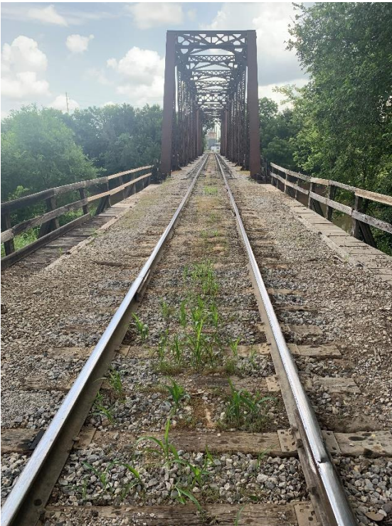
(Moline 247.4-2 Ballast deck Timber approach.)
